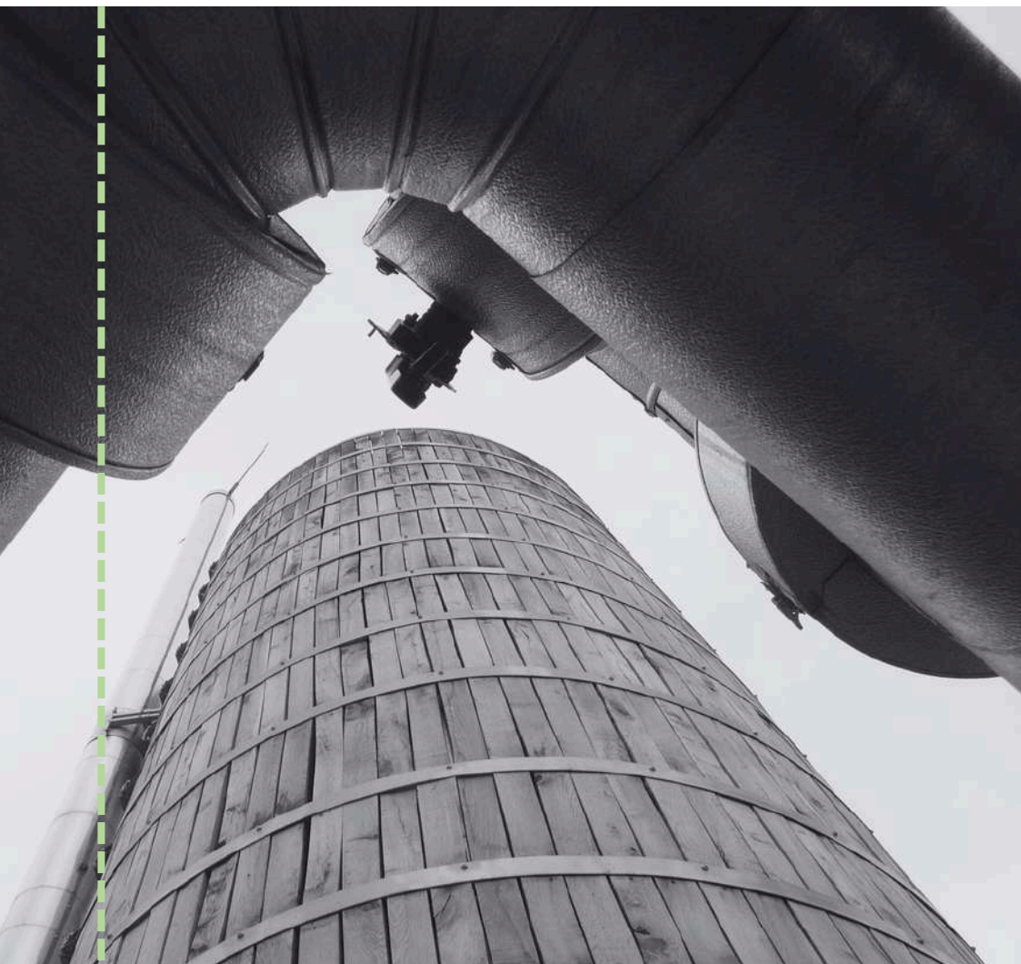
Bunhill Heat and Power Energy Centre
