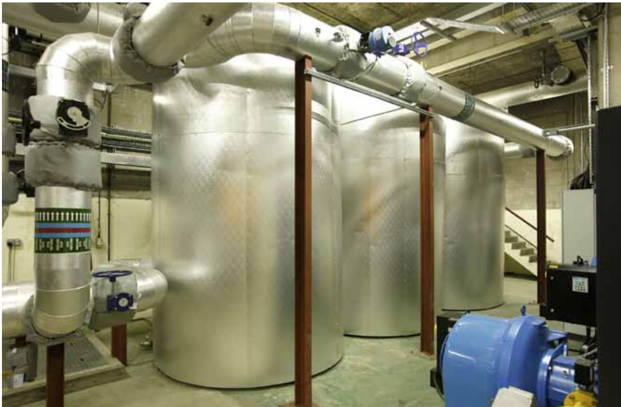
Thermal storage tanks at Riverside Dene, Newcastle.
